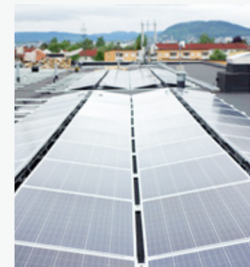
SOLAR PANELS INSTALLED AT NORWAY HEAD OFFICE
