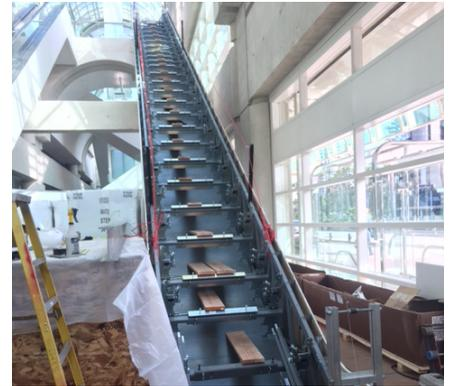
Installation of incline modules is underway on one of the 40-foot units.
