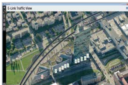
Close aerial view of the building complex layout with equipment
