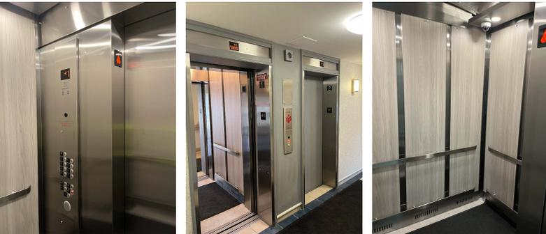
KONE recommended the energy-efficient KONE ReGenerate™ DX modernization package with digital controllers and KONE ReNova™ door operators. Featuring equipment and components produced by KONE, the turnkey solution also improved elevator ride quality for residents at the Winnipeg condominium. "The old elevators didn't level at floors," Johnson says. "Our new ones always level. The noise level decreased, and we've seen a significant reduction in our electrical bills."
